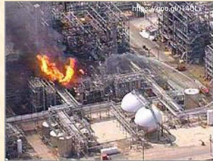
Figure 1. Accident Caused by SIF Failure
