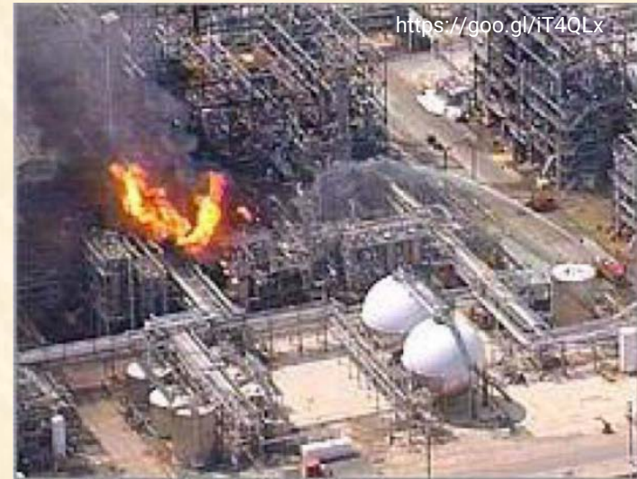
Figure 1. Accident Caused by SIF Failure
