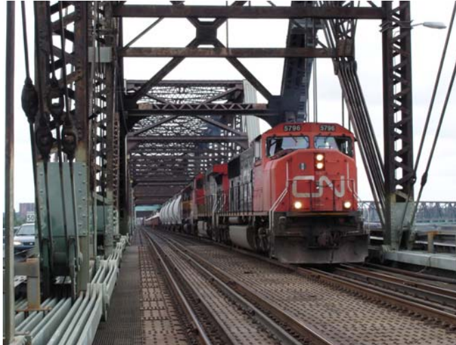
Figure 7. Steel truss bridge instrumented for monitoring study
